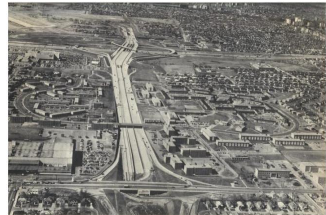
SPADINA (W.R. ALLEN) EXPRESSWAY LOOKING NORTH FROM LAWRENCE AVENUE WEST, STILL UNDER CONSTRUCTION SOUTH OF LAWRENCE IN 1969
