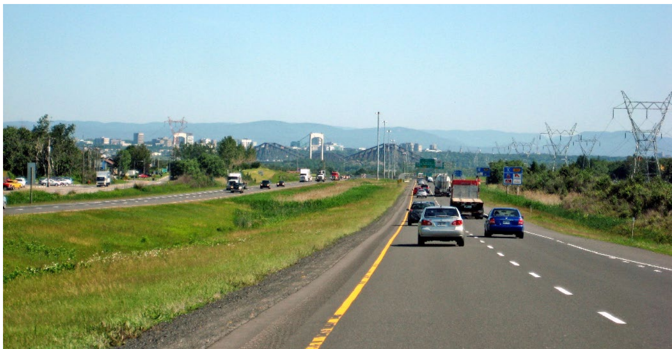
Autoroute 20 est, km 310. Photo: Bobby Hidy [CC-BY-SA-2.0 ( https://creativecommons.org/ )]
